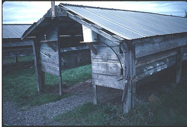
Figure 5. Front of a barn with the float tank feeding the automatic watering system running along the outside of the barn on the back of the cages.
